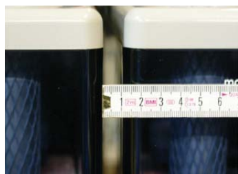
Fig. 5-13: 10 mm clearance between the batteries
