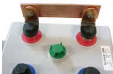
Fig. 5-18: Installing the end terminals (connection plates)
