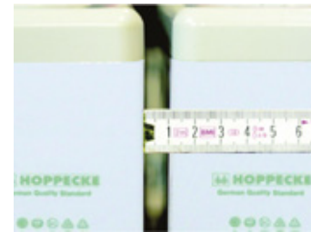
Fig. 5-14: 10 mm clearance between the batteries
